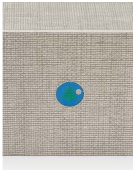
Typical Q-Mark 3rd party fire door identification
