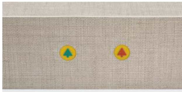
Option 5 - Yellow outer / Green inner Yellow outer / Orange inner Intumescent in door fitted by manufacturer. Glazing by manufacturer.
